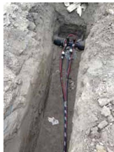
Further benefits included resistance to corrosion. The soils in the area being organic corrosive soil material called “Blue Loom”, PE-4710 HDPE materials eliminate these corrosion factors, which adds to expected life cycle of the pipe line. The home owner’s assessment costs were reduced by half from the Phase I project making hook-ups to the main service more affordable.
