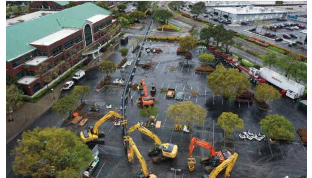
Figure 2: Fused 32-inch diameter PE4710 pipe string on rollers being pulled to borehole
