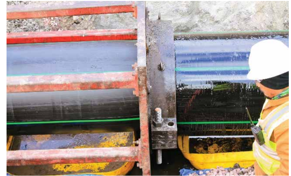
Figure 2: 36-inch HDPE pipe is pulled through a reduction die before entering 36" DI host pipe
