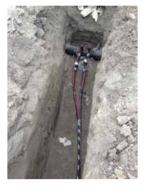
Further benefits included resistance to corrosion. The soils in the area being organic corrosive soil material called "Blue Loom", PE-4710 HDPE materials eliminate these corrosion factors, which adds to expected life cycle of the pipe line. The home owner's assessment costs were reduced by half from the Phase I project making hook-ups to the main service more affordable.
