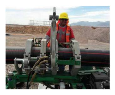
(200psi), with a special printline showing BMW SLP Plant. The potable water system includes a 350,000 gallon capacity tank distributing drinking water. This application involved the installation of 8,628 meters of 1", 2", 6", 8" and 10" High Density Polyethylene DR9, NSF61 blue-striped pipe (200psi), with a special printline showing BMW SLP Plant. The gray water system includes a 350,000 gallon
