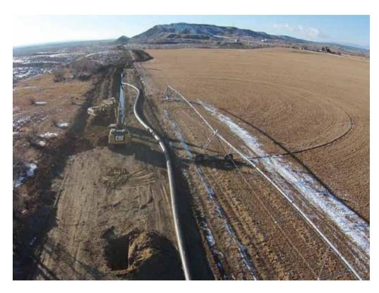
from DR7 to DR32.5, including over 30,000 feet of 30" IPS DR13.5 pipe. PSI's for the project ranged from 10 psi to 300 psi. And with long stretches of open country to cover, runs of 2,000 to 3,000 feet at a time were fused and installed in the trench.
