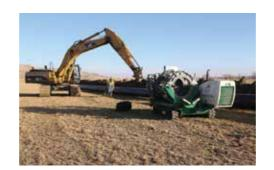
HDPE also eliminated the need for costly fittings and cut down on installation time due to narrower trench widths than those required for other piping materials.
