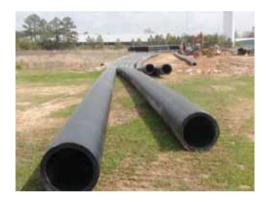
During installation Ken Downey, Superintendent of Installation for JS Haron commented that HDPE pipe provides toughness, durability and flexibility for his installations. This allows him to pre-assemble large sections of the line in a central staging area and move them into position for installation. This saves time and money as well as creating project scheduling versatility, especially when weather conditions are not favorable for HDD or trenching.
