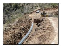
development of the system, WL Plastics provided over 64,000 feet of 4 to 14 inch pipe. The district has been using HDPE pipe for many years, the first installation being the Sky Ranch Pipeline main feed line, back in 1990's. They have been using HDPE pipe ever since then for most of their applications. The district
